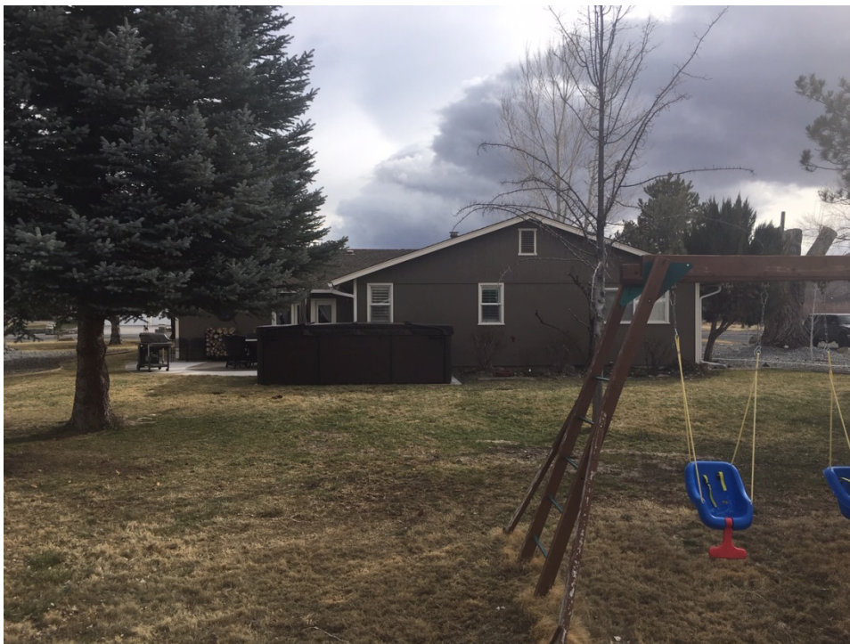
Main Residence – North Elevation
