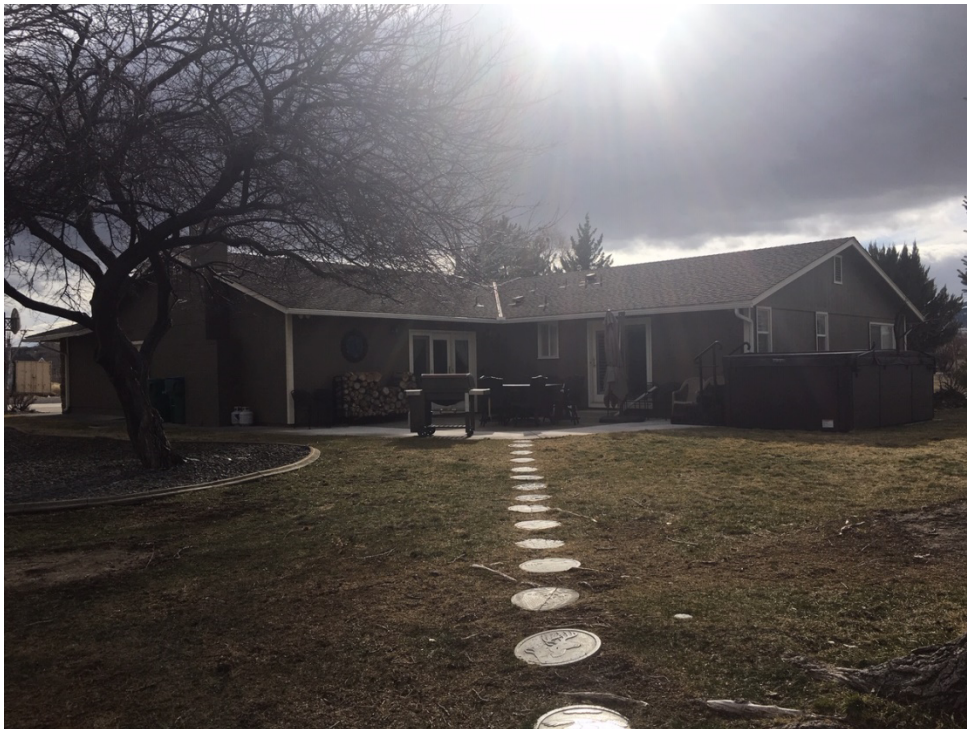
Main Residence – North – East Elevation
