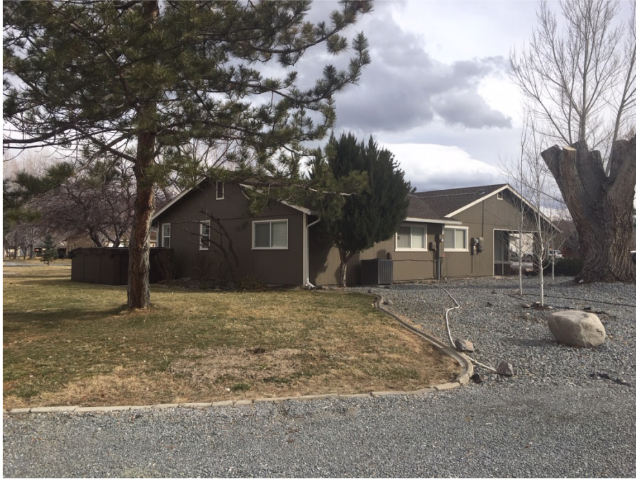
Main Residence – North – West Elevation
