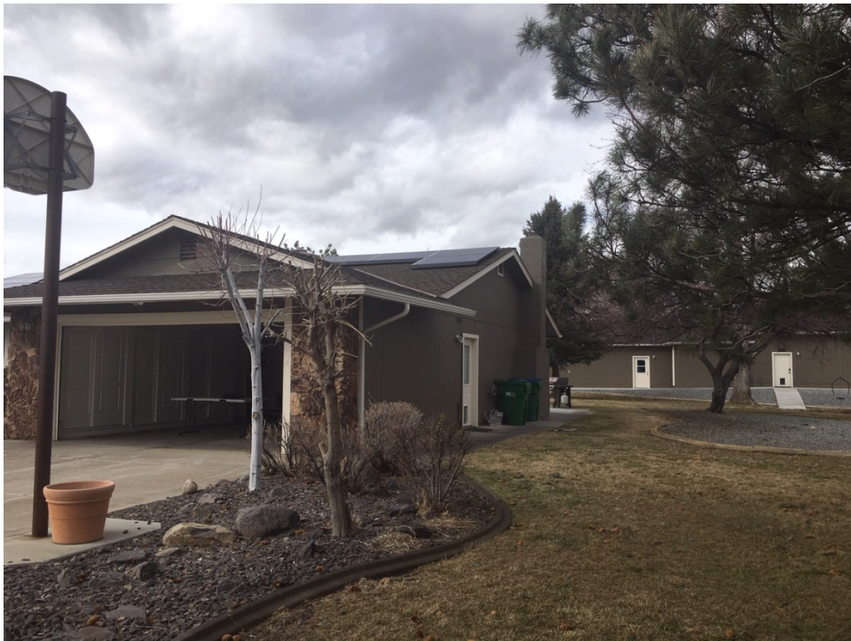
Main Residence – South-East Elevation
